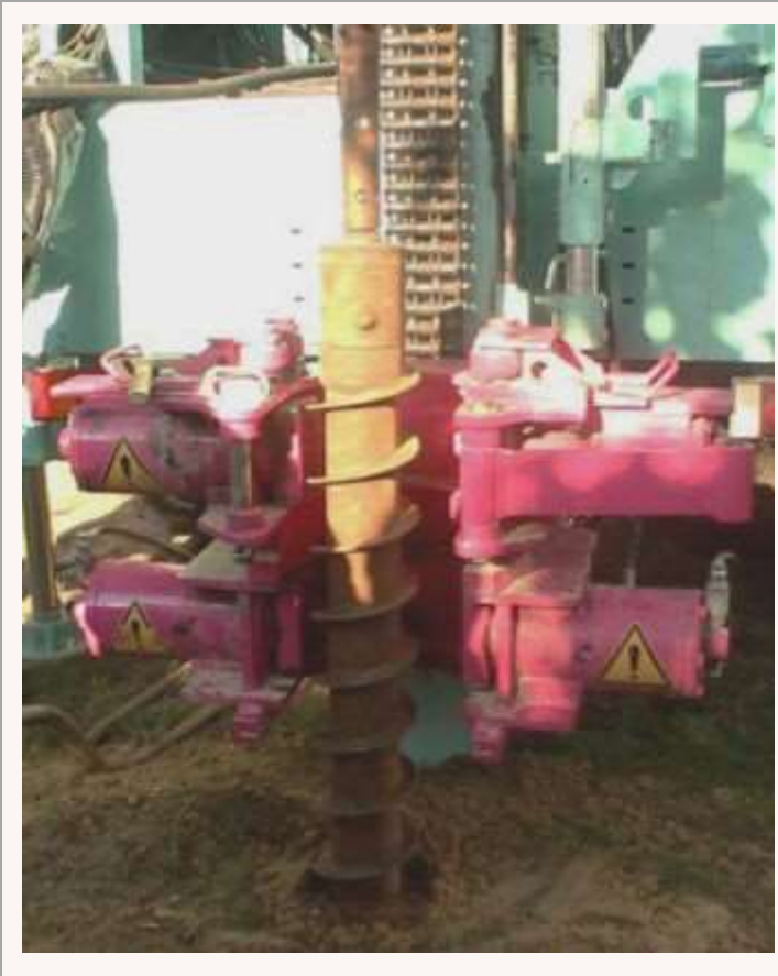
Hollow Stem Auger Drilling
